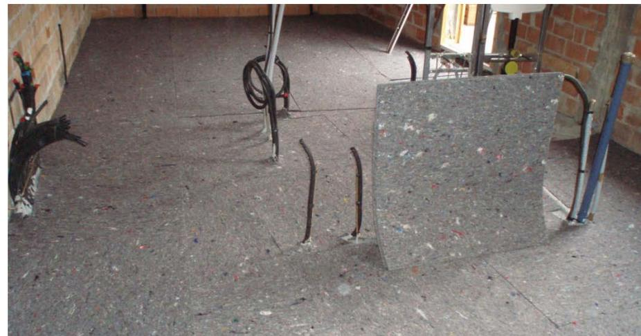
Photovoltaic system - TNT underflooring above systems
